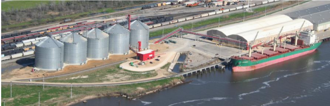
Figure 47: Existing Wood Pellet Silos and Loading Equipment at Port Arthur
