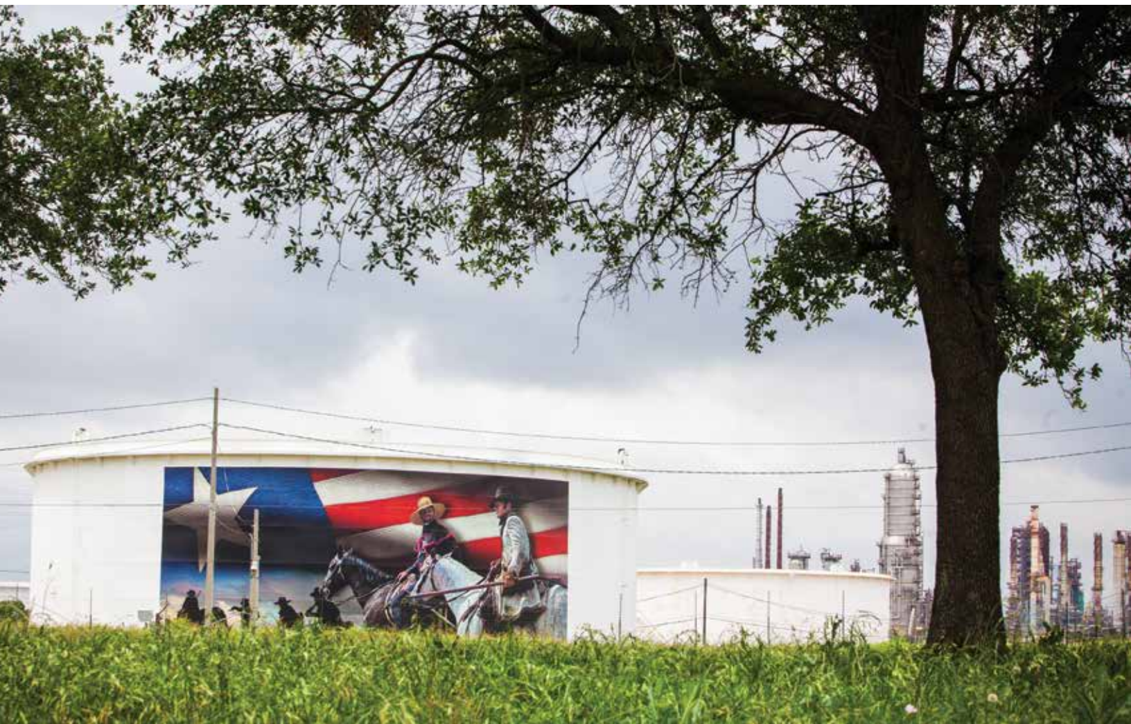
OIL STORAGE TANKS are ubiquitous in the Houston area. Some have murals depicting famous people and events in Texas history. The petrochemical plant in the background is one of dozens in the area.
